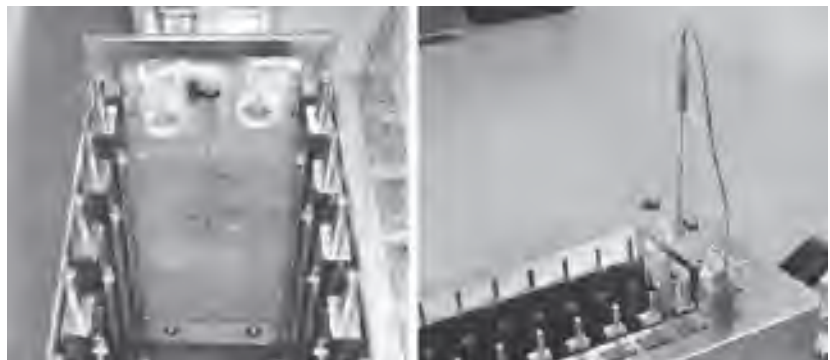
Figure 24: Celsius ® -Pak Placement and Thermocouple Connection
